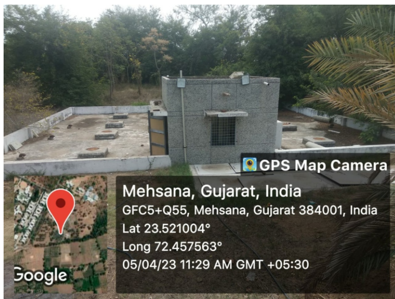
Photos of STP at GUNI Campus
